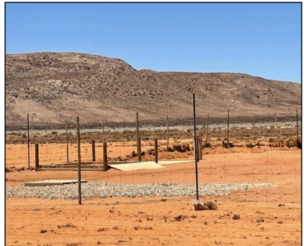
The concrete bund where fuel was stored must be removed and the area rehabilitated
