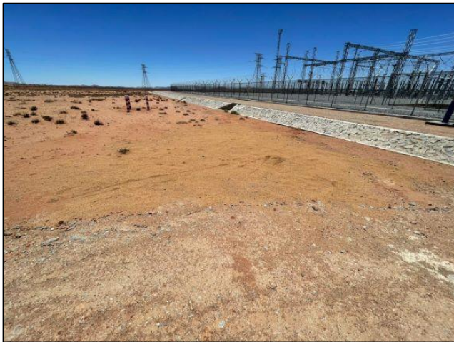
Formalised open stormwater channel adjacent to the substation
