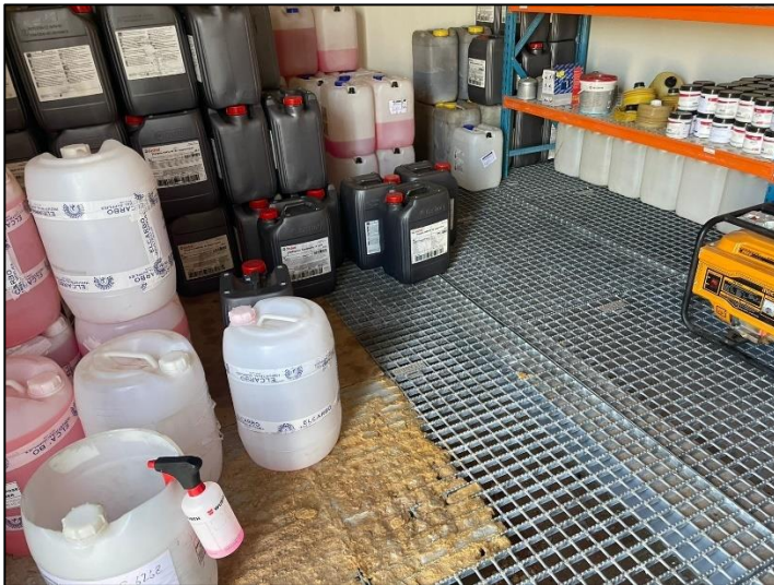
7. Hazardous substances / chemical store fitted with bundled floor to capture any spills / leaks
