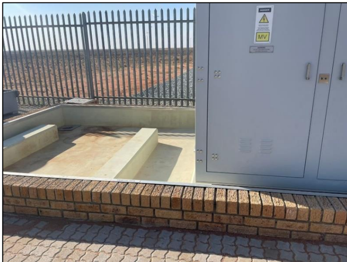
11. Bunded areas around all infrastructure that has the potential to impact the environment
